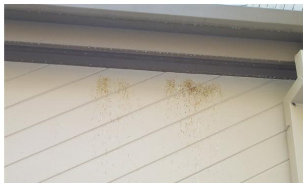
Figure 3. Carpenter bee staining on siding below the fascia.
